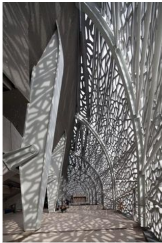
Concrete latticework designed by architect Rudy Ricciotti and made of our Ductal concrete
