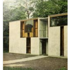
Margaret Escherick House by Louis Kahn. Chestnut Philadelphia. From House Garden, October 1962.
