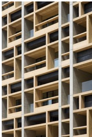
Japanese timber structure, Shinkenchiku-sha
